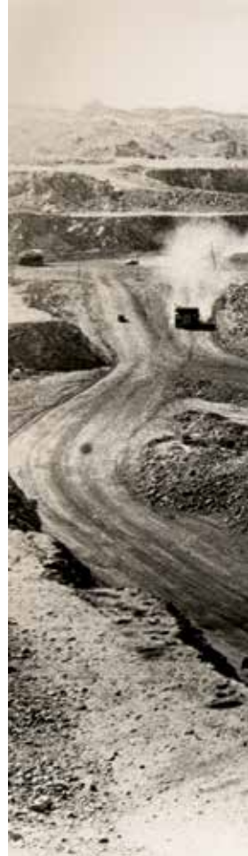
The open pit after the first ten years.
