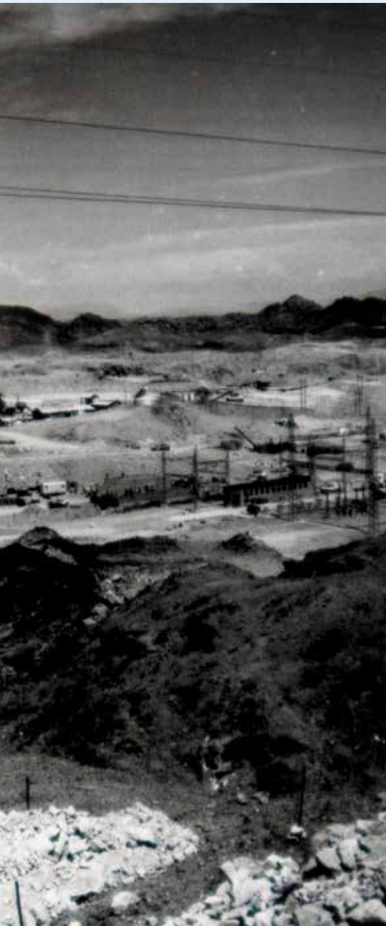
The open pit in the early years. Today, known as the SJ Pit, it currently measures at 3.5 kilometres in length, 1.5 kilometres in width and 420 metres in depth.
