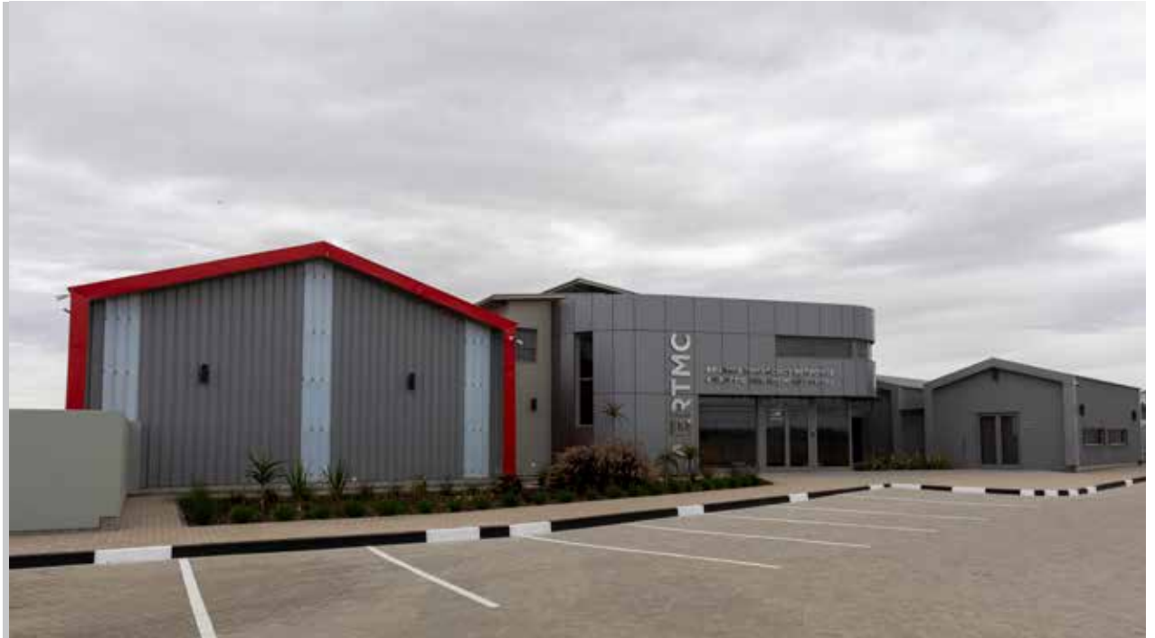
The Arandis Emergency Response and Traffic Management Centre.
