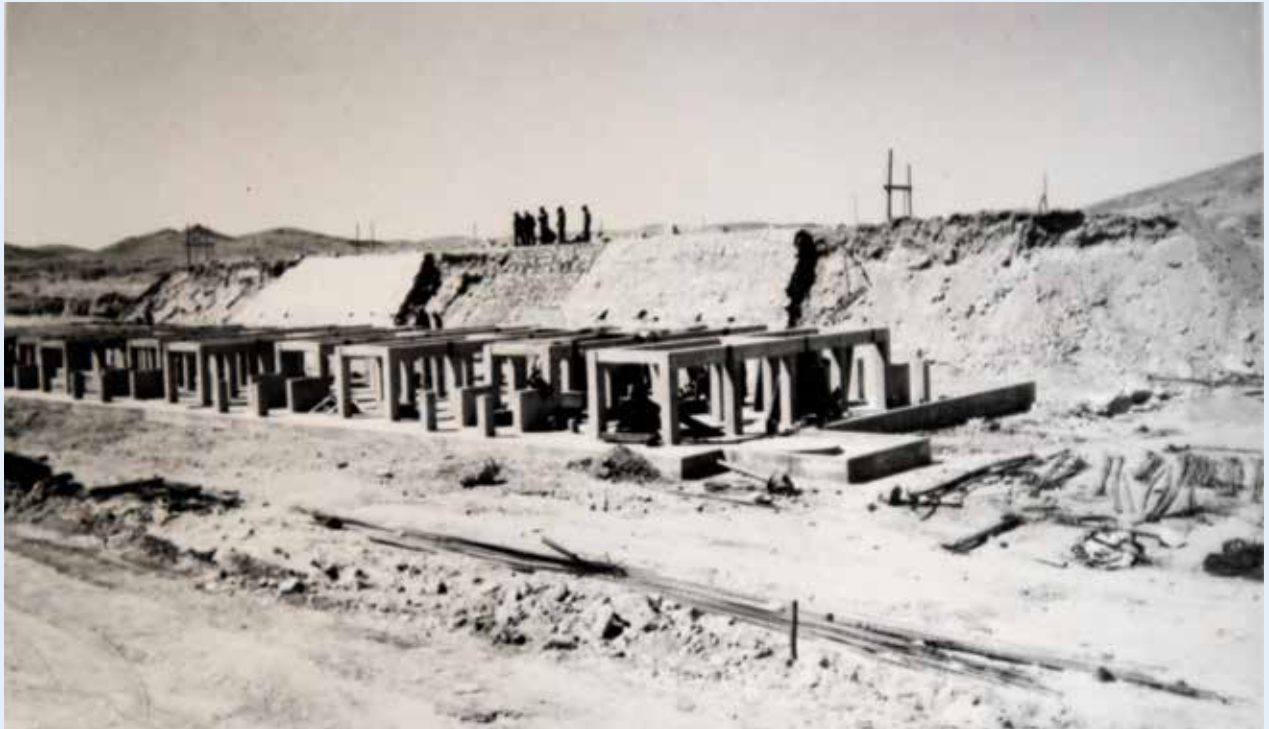
Early buildings and railway line of the mine's construction phase.
