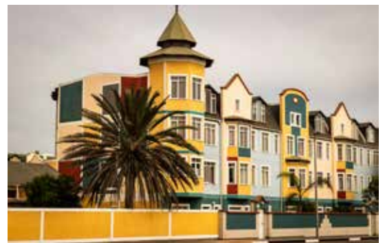
A modern townhouse complex, continuing the German colonial architecture.
