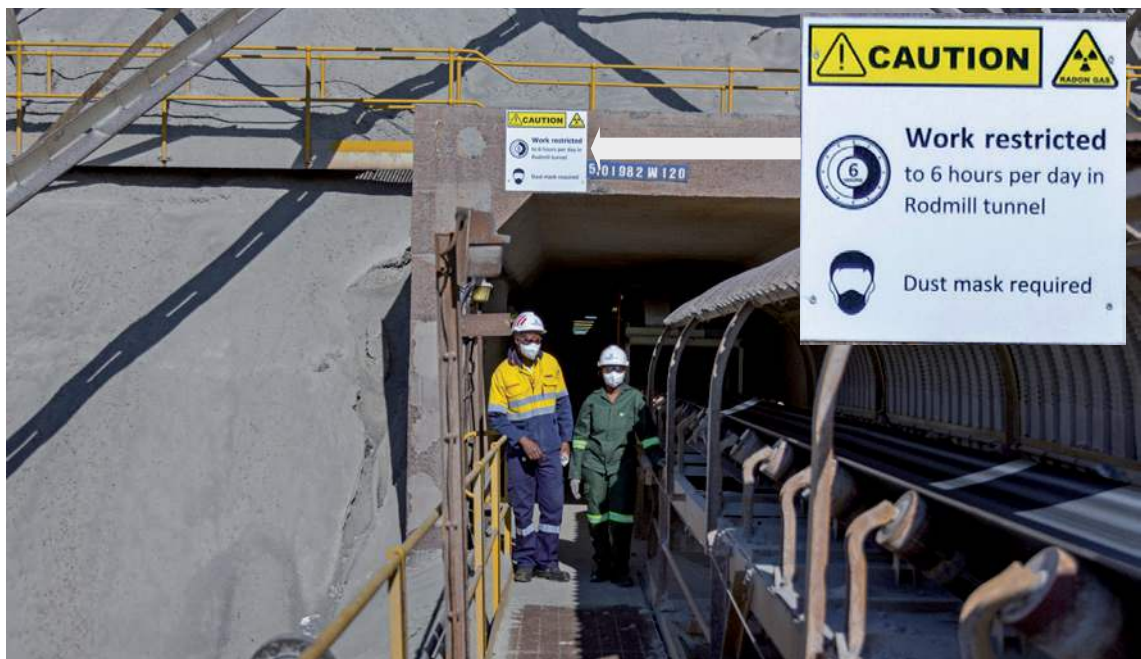
Figure 9: Rod mill tunnels with time restriction signage.
