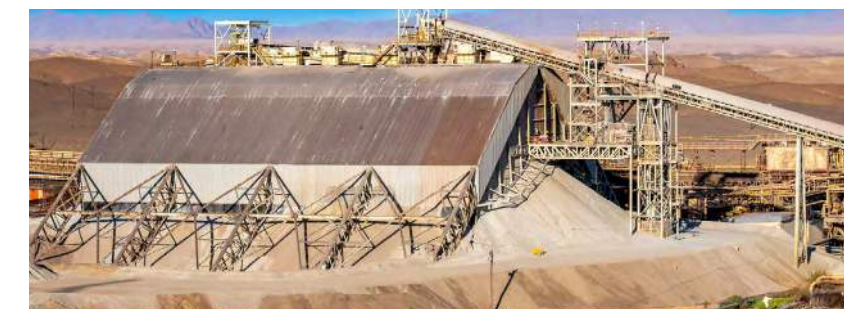
Through a multi-unit operation process of crushing, grinding, leaching, continuous countercurrent decanting, ion exchange, solvent extraction, precipitation, calcination, CNNC effectively dissolved and extracted the uranium in ore to produce high quality uranium octaoxide (U 3 O 8 ) products
