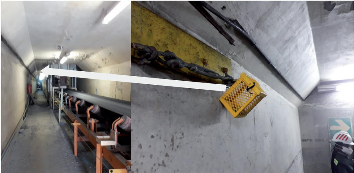
Figure 8: A rod mill tunnel (left) – the arrow shows the location of the monitoring equipment close to rear of tunnel.
