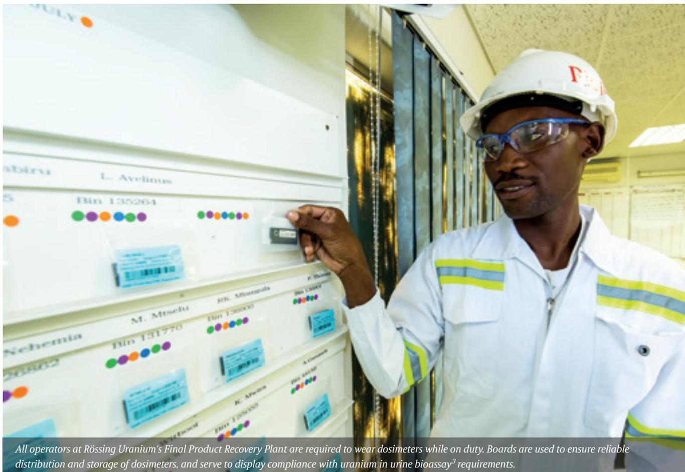
All operators at Rössing Uranium's Final Product Recovery Plant are required to wear dosimeters while on duty. Boards are used to ensure reliable distribution and storage of dosimeters, and serve to display compliance with uranium in urine bioassay<sup>3</sup> requirements.
