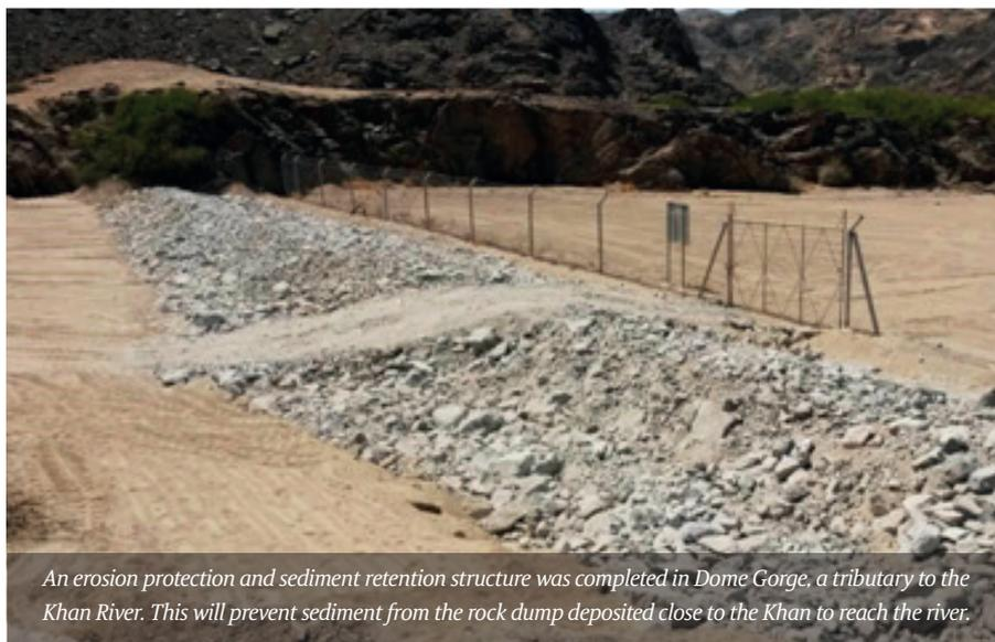
*An erosion protection and sediment retention structure was completed in Dome Gorge, a tributary to the Khan River. This will prevent sediment from the rock dump deposited close to the Khan to reach the river.*
