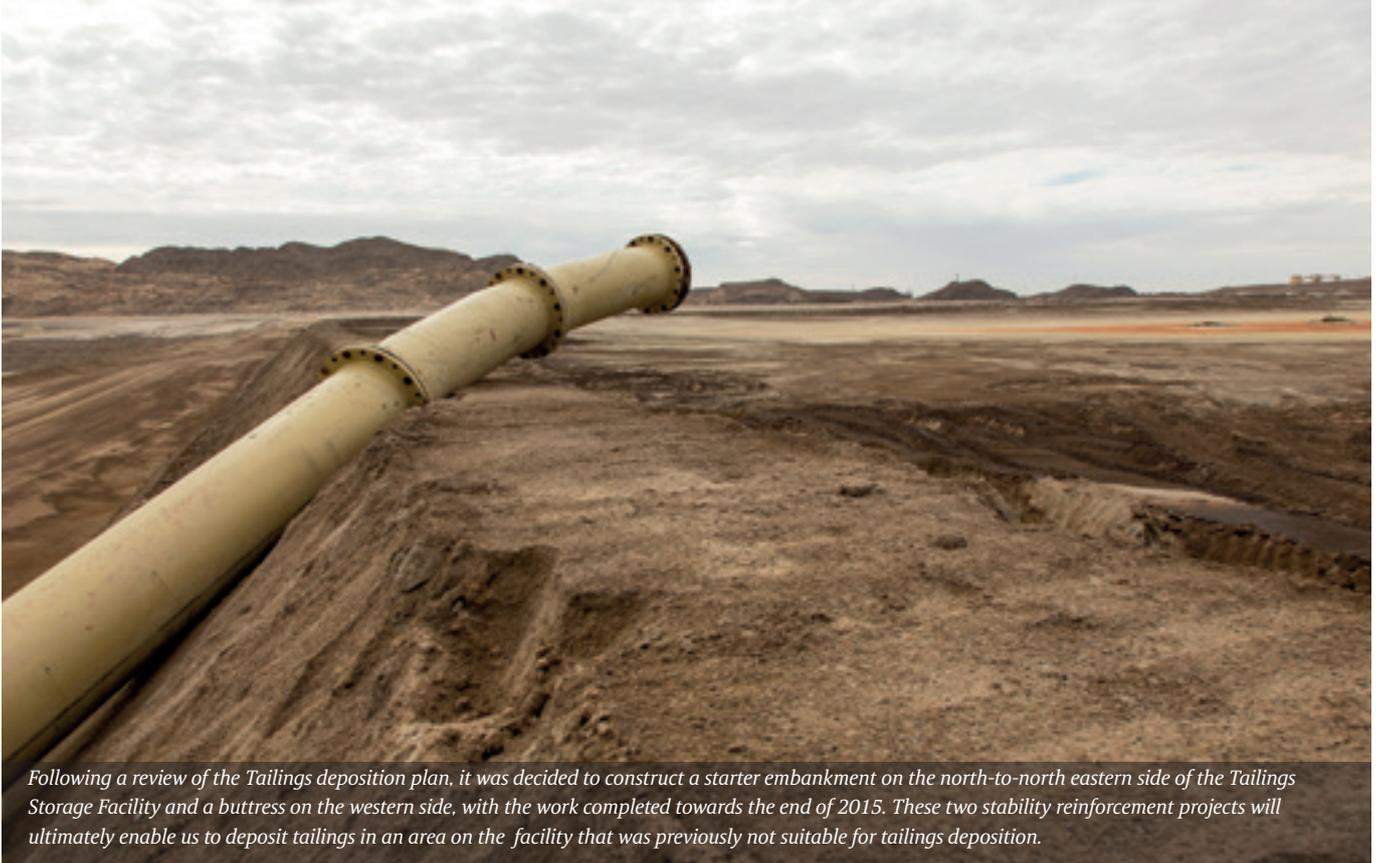
*Following a review of the Tailings deposition plan, it was decided to construct a starter embankment on the north-to-north eastern side of the Tailings Storage Facility and a buttress on the western side, with the work completed towards the end of 2015. These two stability reinforcement projects will ultimately enable us to deposit tailings in an area on the facility that was previously not suitable for tailings deposition.*
