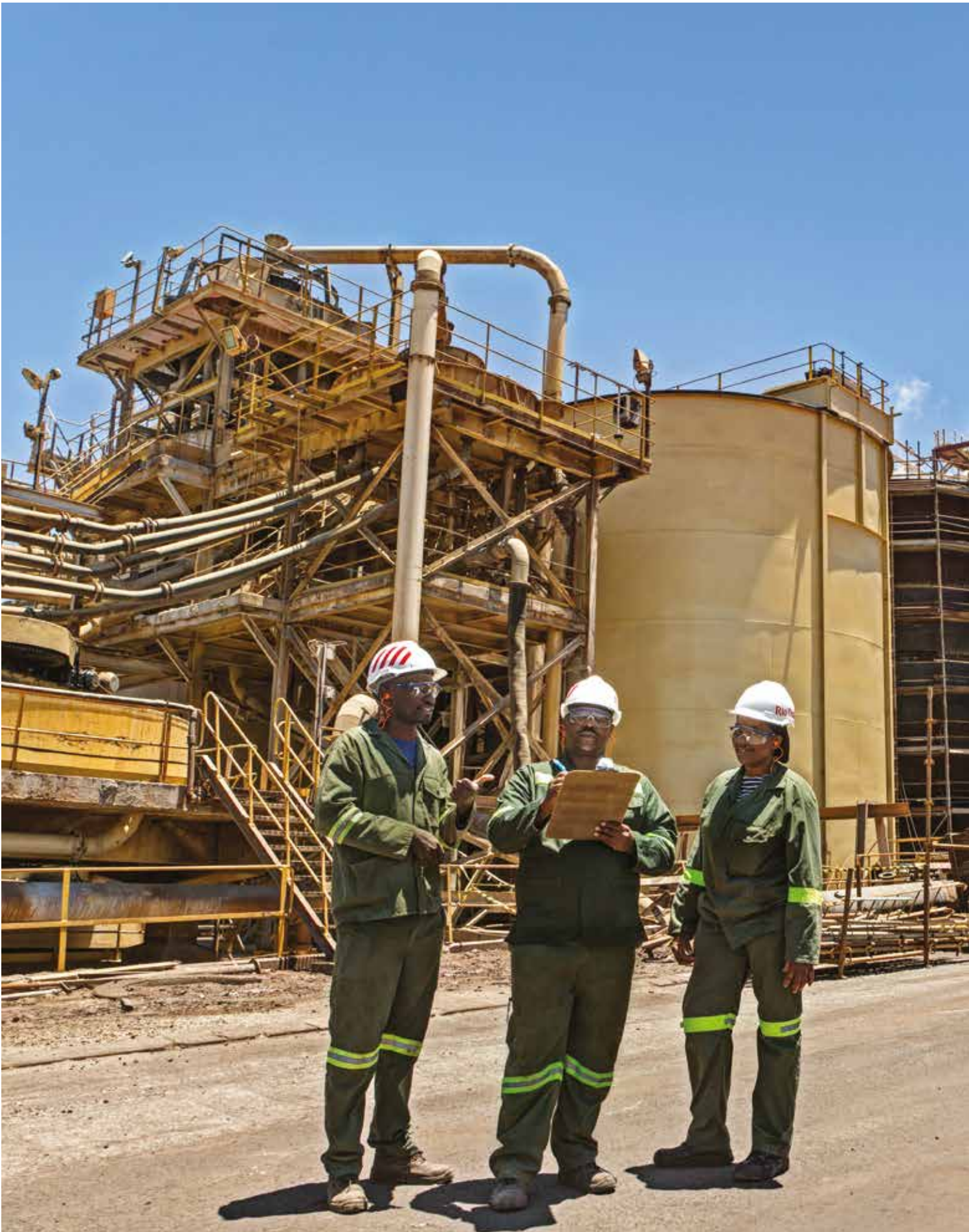
The refurbishment of the leach tanks is part of a ten-yearly refurbishment programme to ensure that the structure of the leach tanks is in good condition. Risk assessments are carried out by the workers to check that the work is carried out safely. Employees of the Namibian Engineering Corporation (NEC), Sam Nujoma, Stephanus Mouton and Teopolina Fanuel are conducting a safety check while working on the refurbishment of one of the leach tanks.
