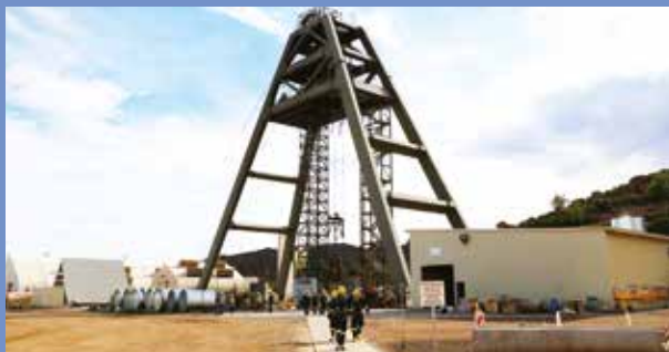
The A-frame over Shaft 10 at the Resolution Copper project outside Phoenix, Arizona, US.
