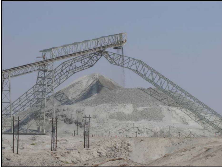
Figure 4-11: Coarse ore stockpile.
