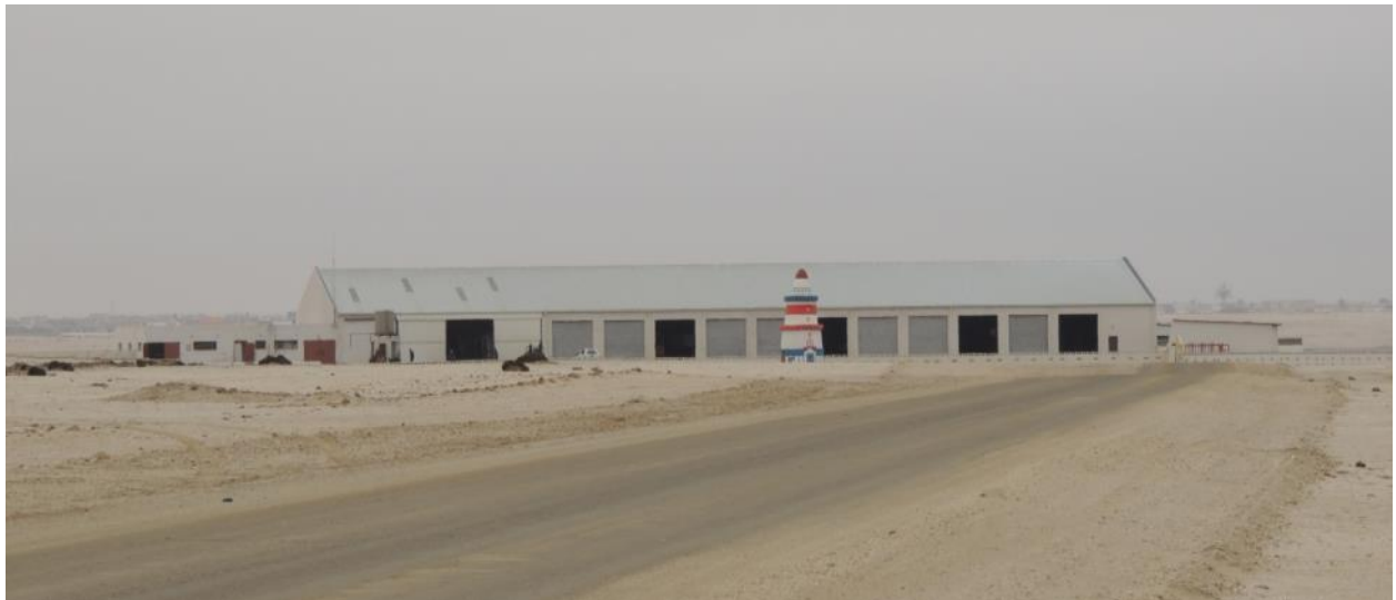
Figure 37: Photograph depicting the existing Salt Company (Pty) Ltd structures and salt stockpiles and warehouse
