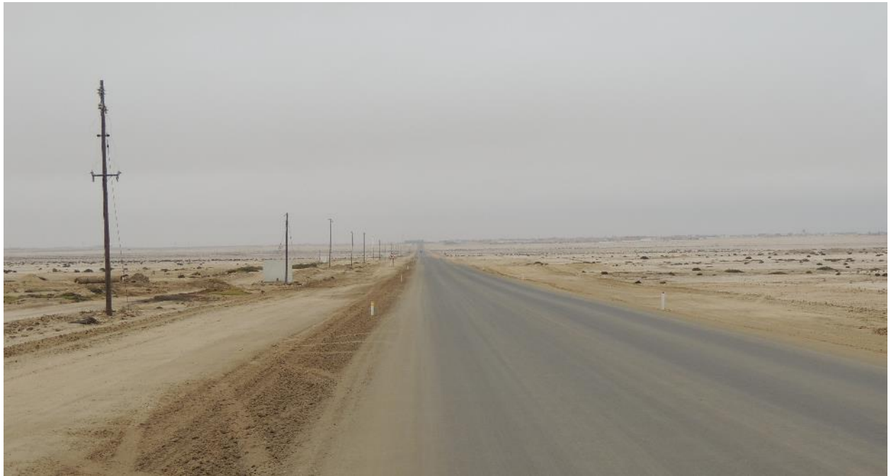
Figure 36: Photograph taken south of the C34 National Road with Swakopmund town in the background
