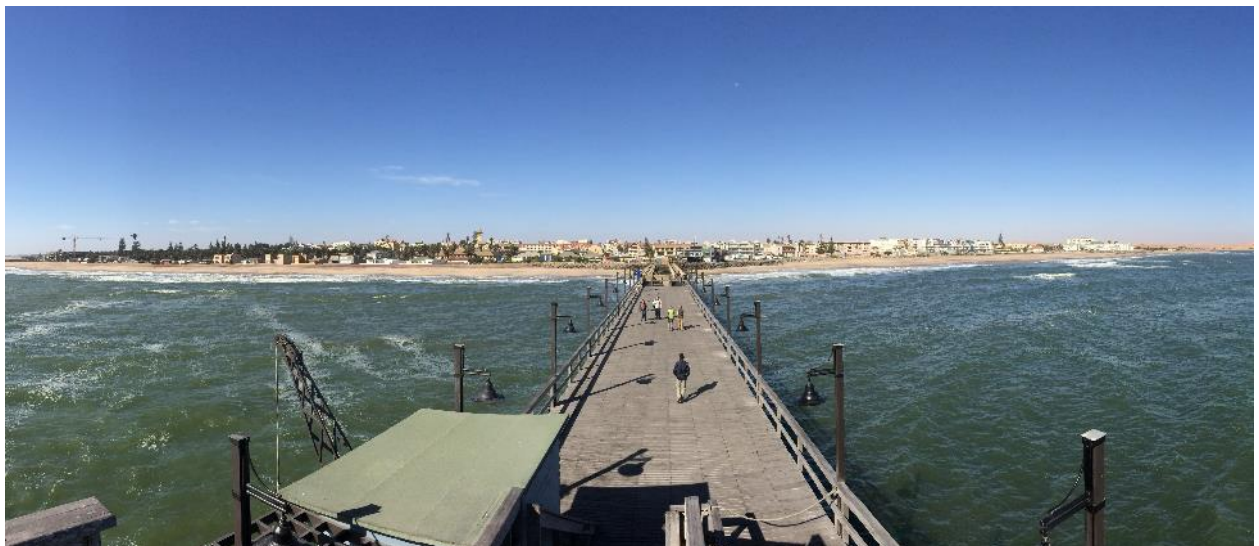
Figure 35: Panoramic photograph of Swakopmund town from the renowned Jetty south of the main beach
