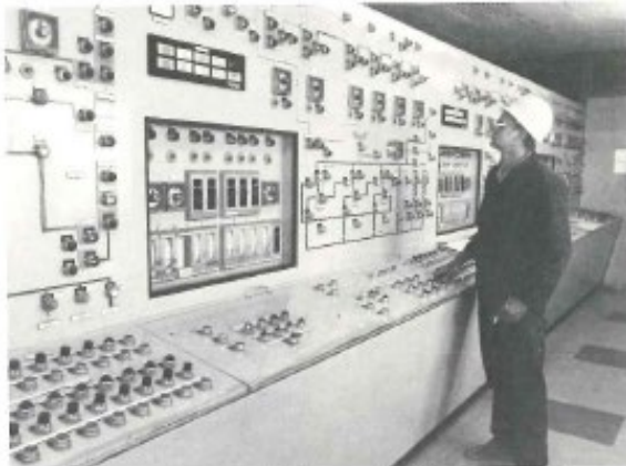
The old CIX control - before CPC. CPC was only commissioned in 1983.
