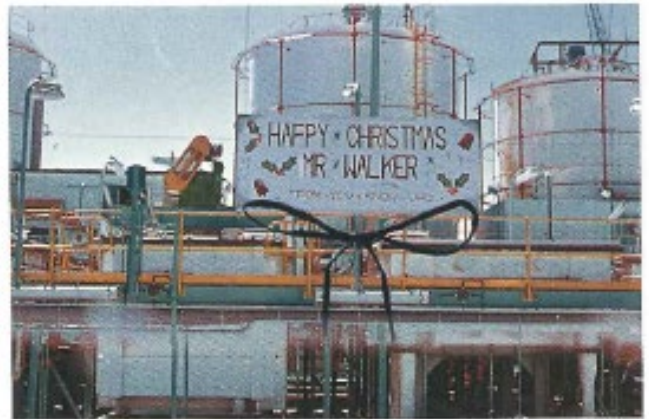
Half of the SX plant had to be rebuilt after a fire broke out at midnight on 24 May, 1978.
