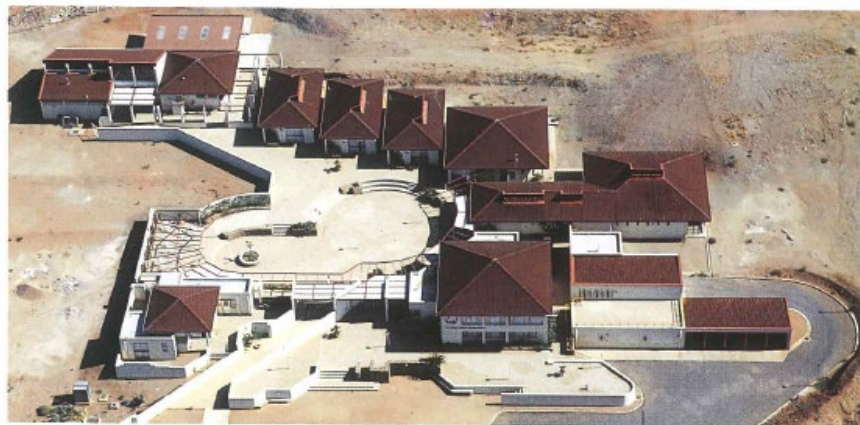
Aerial view of the Rössing Foundation Adult Education Centre.
