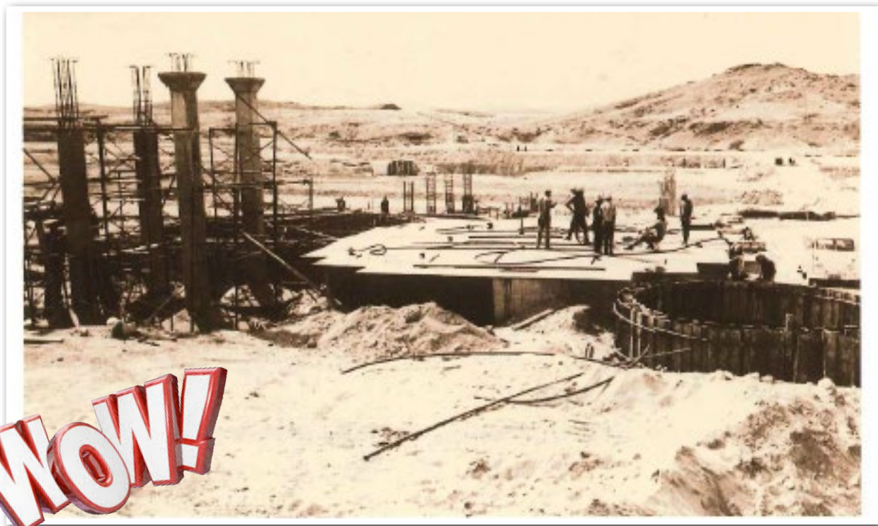
Believe it or not, but this photo shows the erection of our Processing plant's leach tanks - in April 1975!
