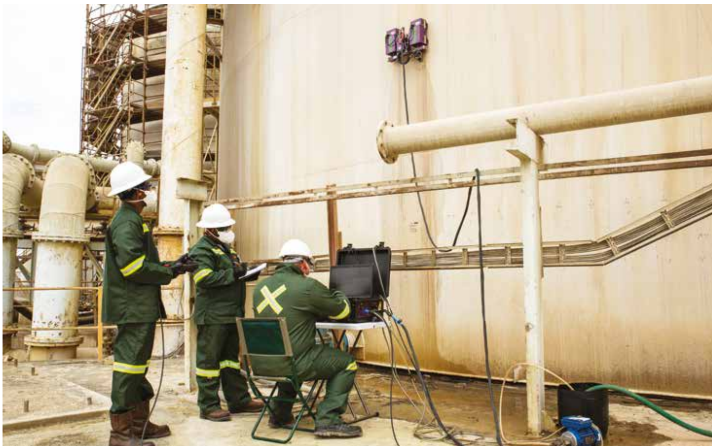
A rapid-motion scanner was used on storage tanks to evaluate the condition of the tanks' shell thickness. Employees of the contractor, Petro Base, operating the equipment are from left to right Clement Nduka and Ambrose Ezimoha, advanced non-destructive testing specialists, and Johan le Roux, managing director of Petro Base South Africa.
