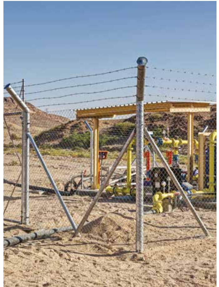
One of the newly-installed seepage recovery points in a tributary of the Khan River, consisting of a well (photo left) and a pump station (photo right). In 2017 we concluded a large scale, intense revision of our water-quality management programme with the outcome of a structural upgrade on the seepage recovery systems, which involved installation of fully automated, state-of-the-art telemetry systems, currently in construction and to be commissioned in early 2018.
