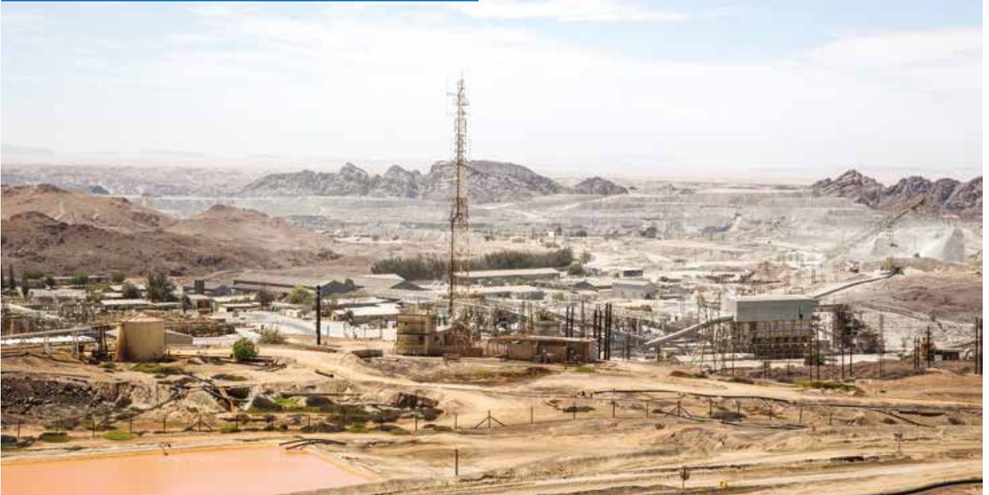
An overview of part of the mine's Processing Plant in the foreground while part of the open pit can be seen in the background.
