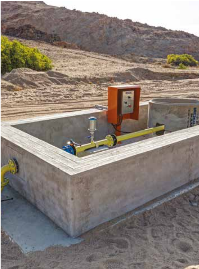
One of the newly-installed seepage recovery points in a tributary of the Khan River, consisting of a well (photo left) and a pump station (photo right). In 2017 we concluded a large scale, intense revision of our water-quality management programme with the outcome of a structural upgrade on the seepage recovery systems, which involved installation of fully automated, state-of-the-art telemetry systems, currently in construction and to be commissioned in early 2018.
