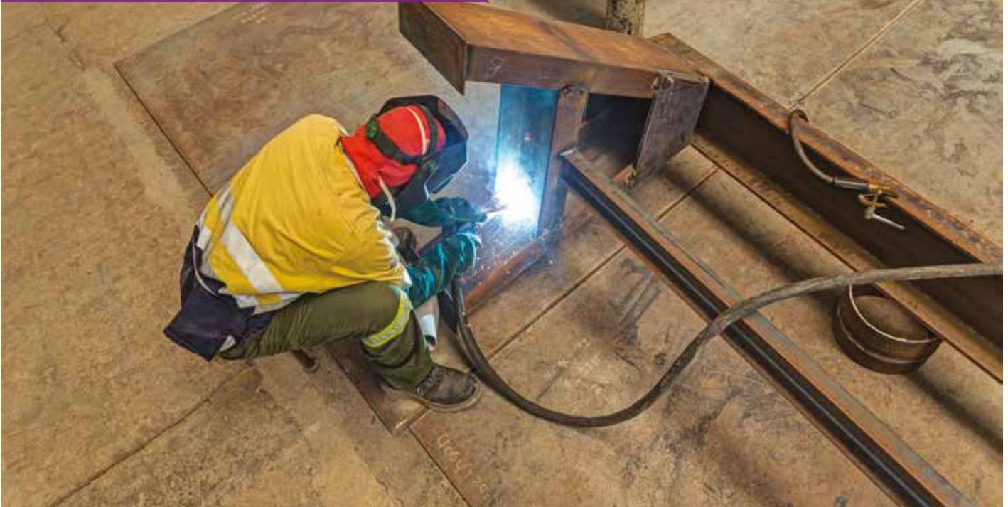
Artisan Elieser John, doing welding work at the mine's plate shop.
