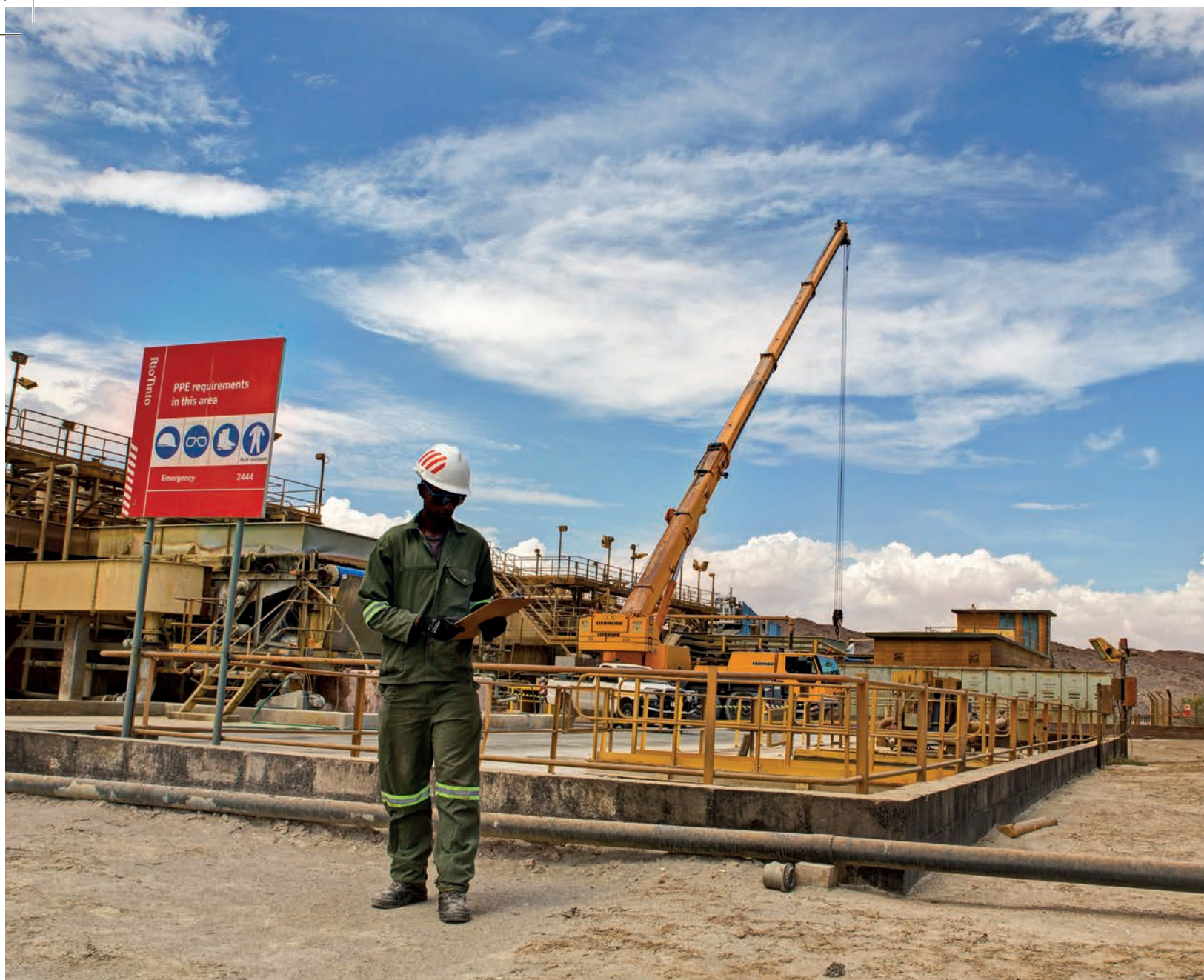
(Above) Safety signage ensures that workers adhere to the specified PPE (Personal Protection Equipment) requirements for each area.
