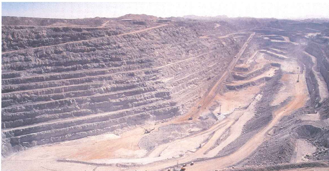
The open pit is 3km long, 1km wide and 300m deep.
