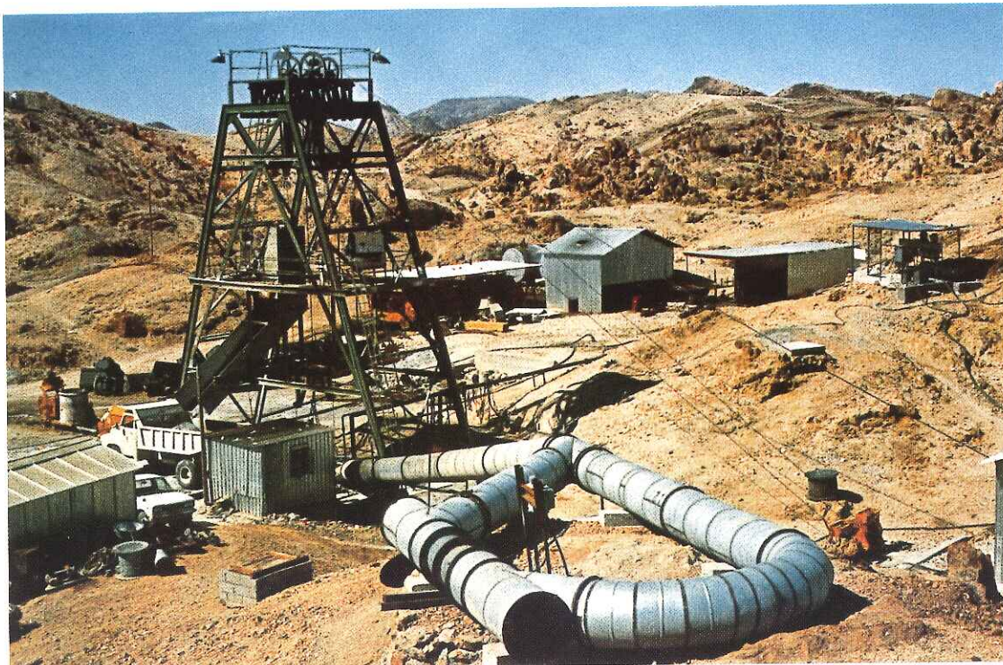
Headgear for the underground pilot operation in the mid-1970's.
