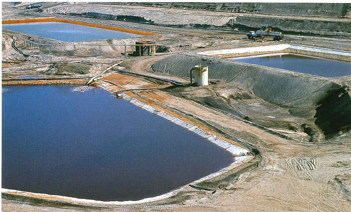
Water from various areas of the plant is collected for re-use
