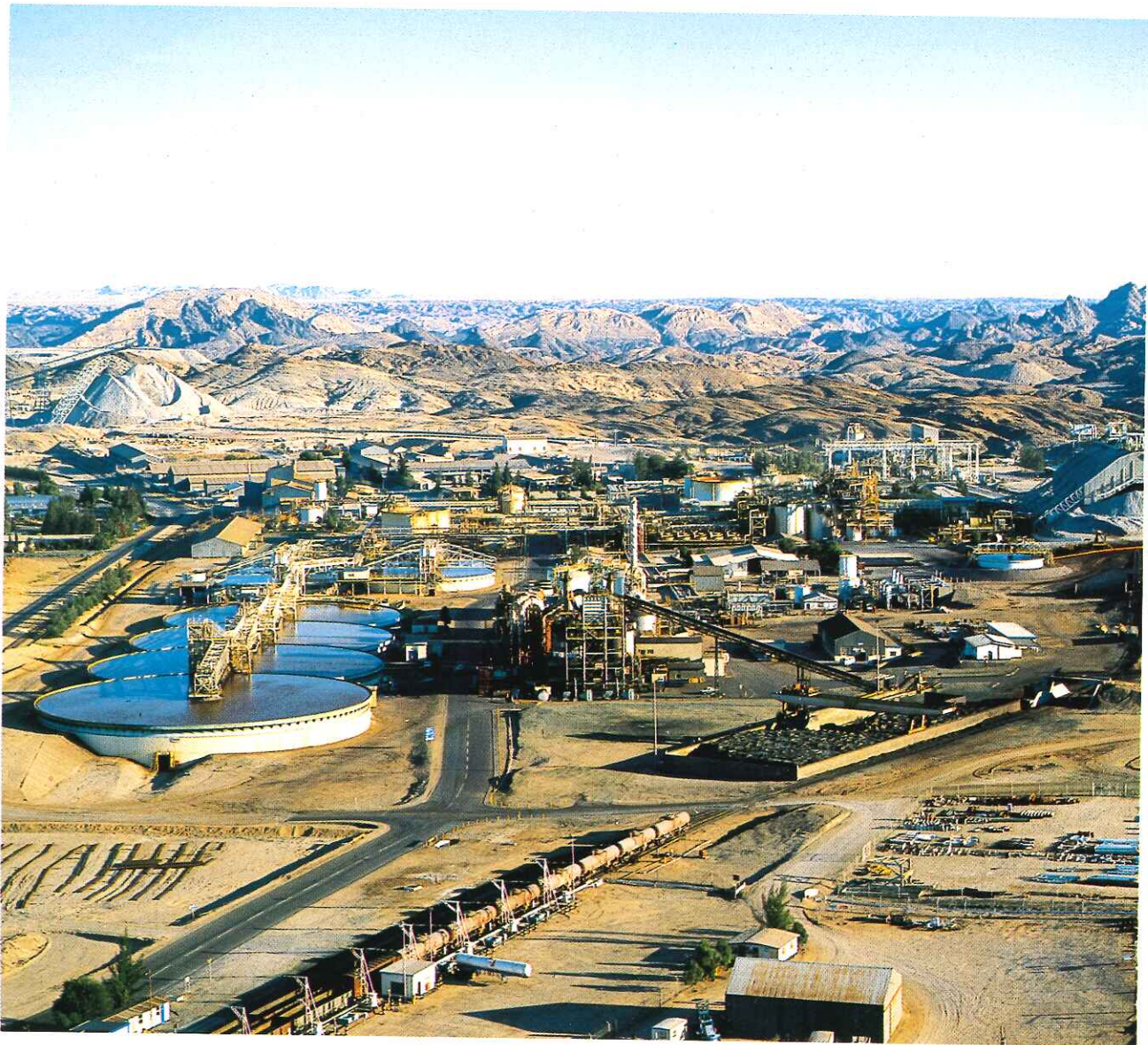
Aerial view of the plant
