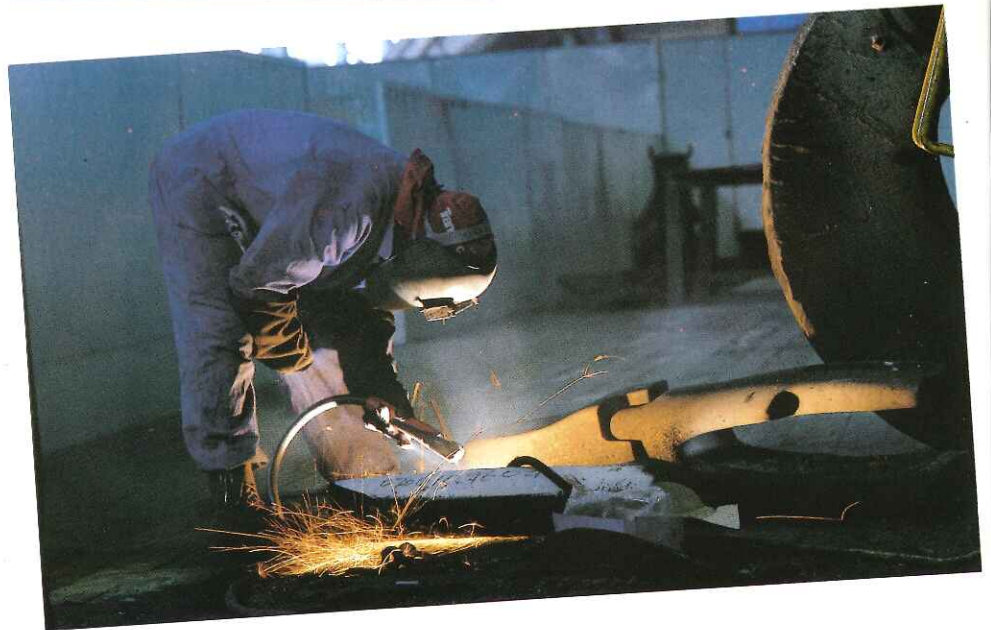
Repairing the bucket tooth of a shovel.
