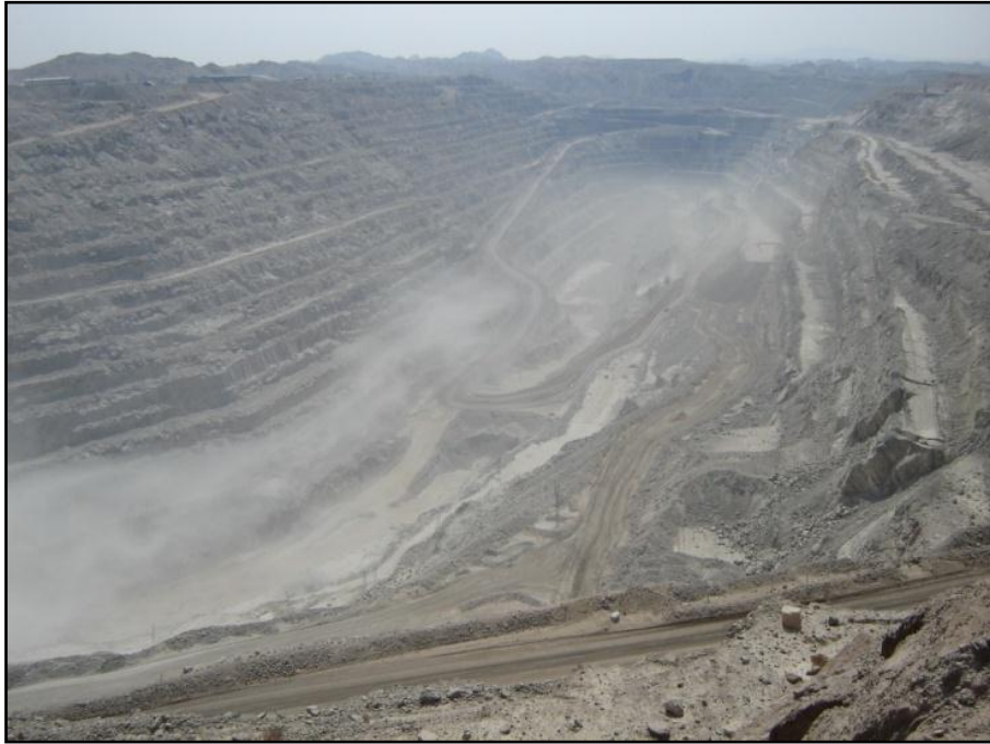
Figure 24: Dust emanating from the pit
