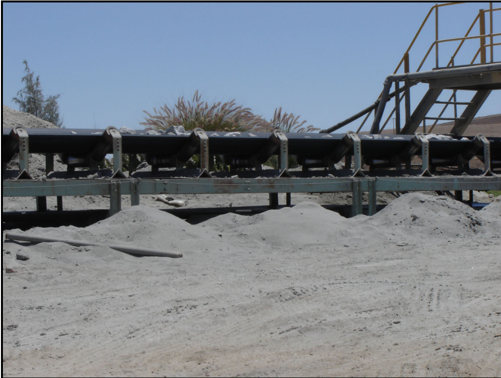
Figure 4-13: Loose material along conveyor belts
