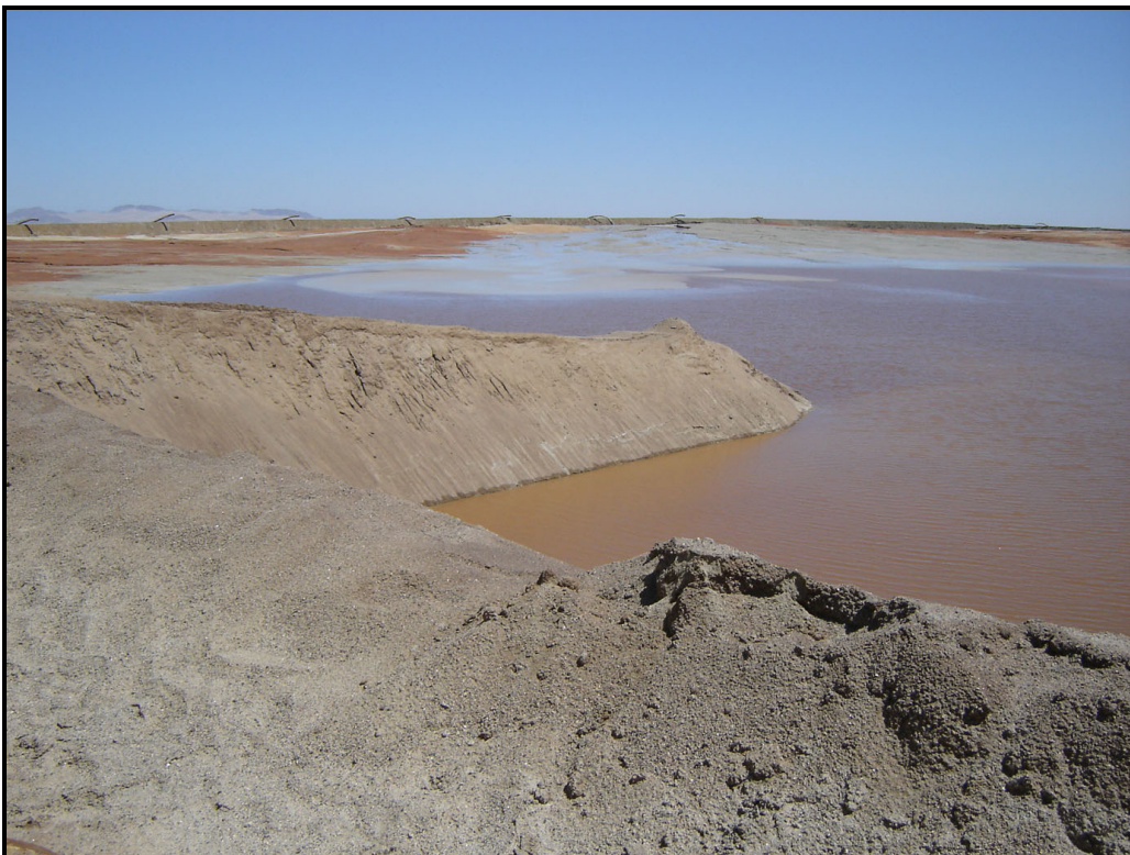
Figure 4-14: Tailings dam at Rössing Uranium Mine
