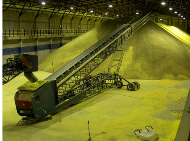
Figure 10: Extendable conveyor for sulphur stockpiling 15
