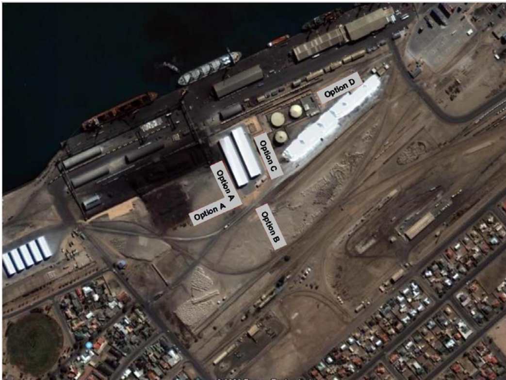
Figure 15: Alternative sites for the sulphur handling facility in the Port of Walvis Bay (source: RU)
