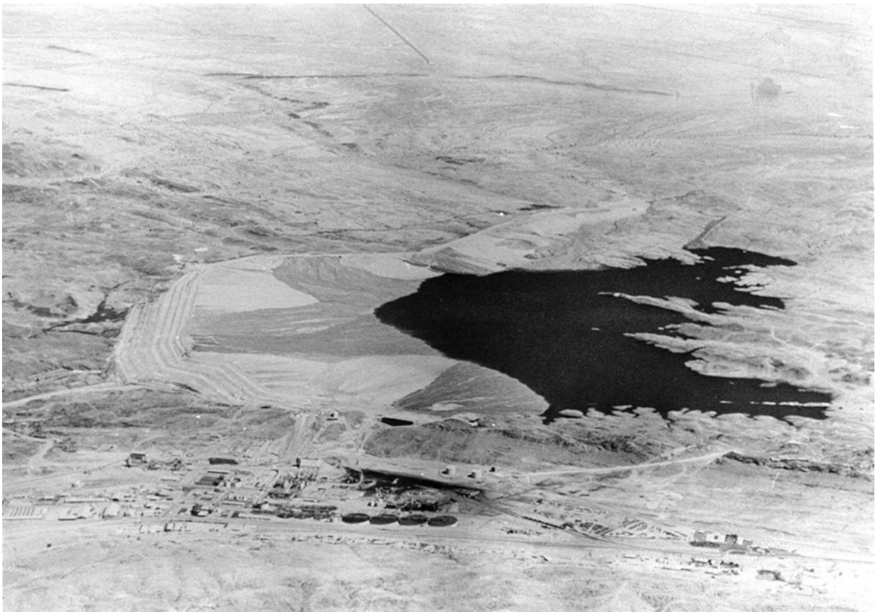
Figure 9: Original tailings dam design of 1982, viewed from the east (source: RU)
