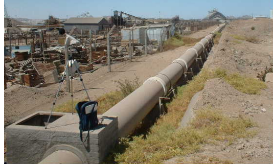
View of pipeline, proposed site to right
