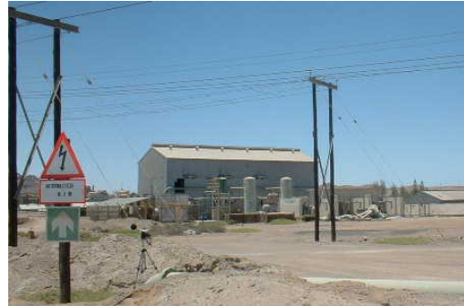
View towards compressor house
