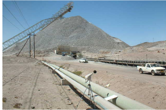
View towards primary reclaim area
