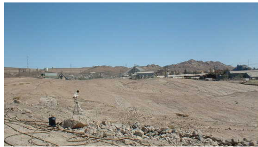
View towards main plant
