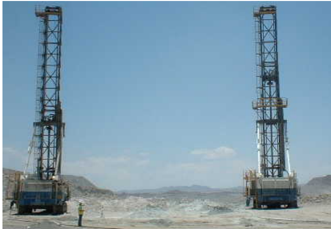
Primary Drilling Rigs
