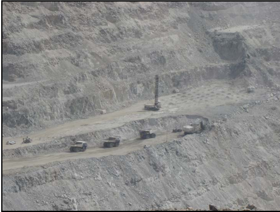
Figure 4-4: Drilling operations in the pit.
