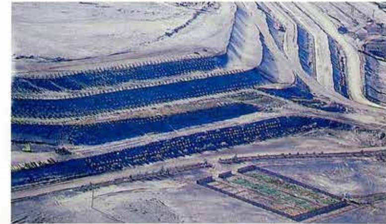
(B) Aerial view of vegetation trial plots on the south-western side of the tailings impoundment.
