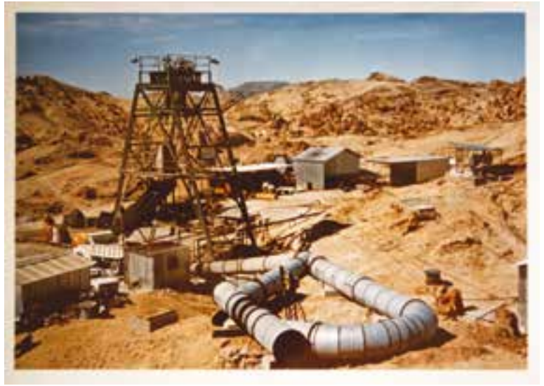
The original vertical shaft that was being constructed near the present day Haultruck Workshop. Rössing started as an underground mine before they discovered that grade was too variable and the ore band widths were too variable for underground mining to be successful.
