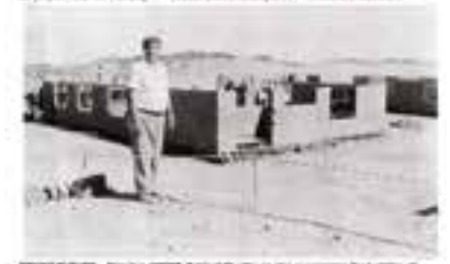
BRICKS FOR THE FUTURE. Director ECKHART Mueller, in Arandis supervising the building of Phase II which started in January this year.
